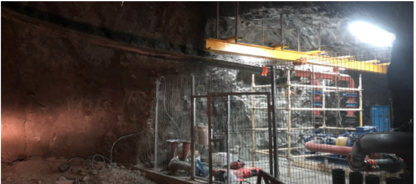
Installation of Pexgol pipes for the drainage of an underground mine
